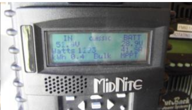
MC250 tracking 1.23 kW MPPT from a PLT80
