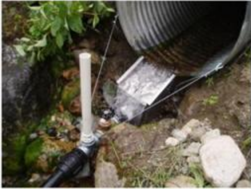
Commercial intake on road culvert
