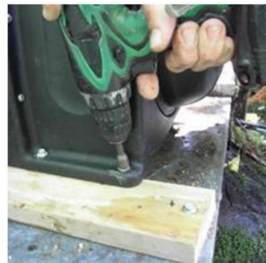
Fixing a turbine to a timber base
