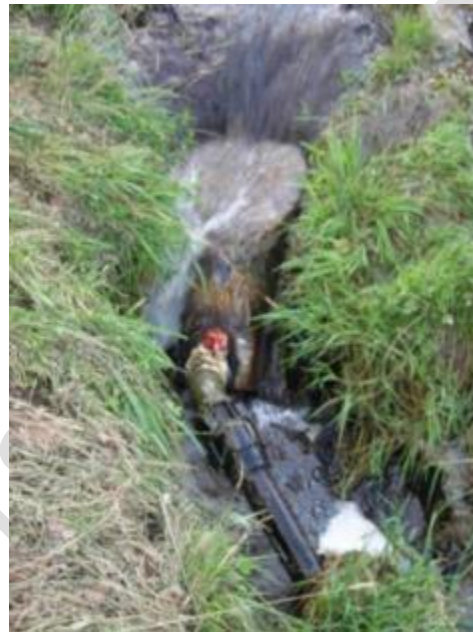
Intake made from stainless steel scrap
