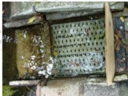
Perforated galvanized cable tray intake
