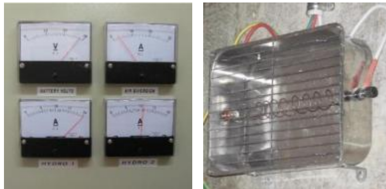
Meter cabinet and resistive load
