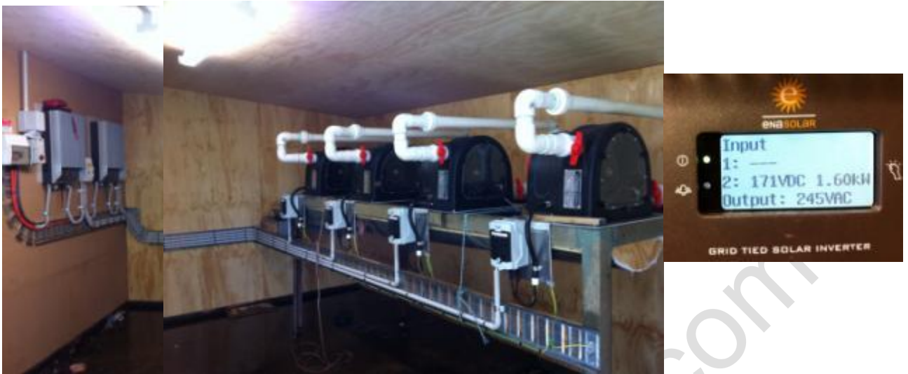
6.4kW from 4 x PLT200's (running at 171 VDC) feeding into 2 x 4kW EnaSolar inverters
