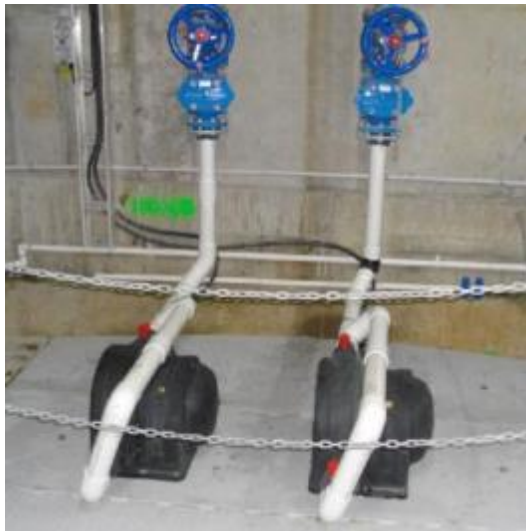
Dual install, one unit runs on 30m (98 ft) head the other 10m (33 ft) head
