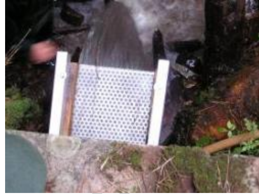
Flat screen in road culvert
